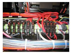
Equipment directly related to chamber operation is controlled within the technician's operation station. If power is lost with equipment related to chamber operation one should first remove upper panels on rear of control panel to view distribution breakers. Control breakers are different from what is found in standard distribution panels. Control breakers are small in comparison and function differently. Each
